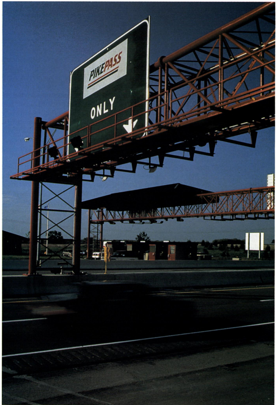
Figure 10. Oklahoma's Pikepass program is an example of electronic toll collection. Pikepass, implemented in 1991 on the state's 478-mile Turnpike system, uses a palm-sized integrated-circuit card mounted behind a vehicle's rear-view mirror. The card responds to a radio beacon emitted by a transmitter beside special Pikepass entry lanes, which are identified by an overhead sign. A charge is automatically deducted from the user's prepaid account. Users need not stop or slow down. Video cameras record license plates of violators. About 100,000 vehicles currently participate, and the revenues collected from Pikepass participants account for almost one-third of Oklahoma's annual toll revenues. Such systems can easily be adapted to vary the toll depending on time of day, as is now done in Norway and will be done in 1995 on privately built express lanes on the Riverside Freeway in California. (Photographs courtesy of Amtech Inc.)
