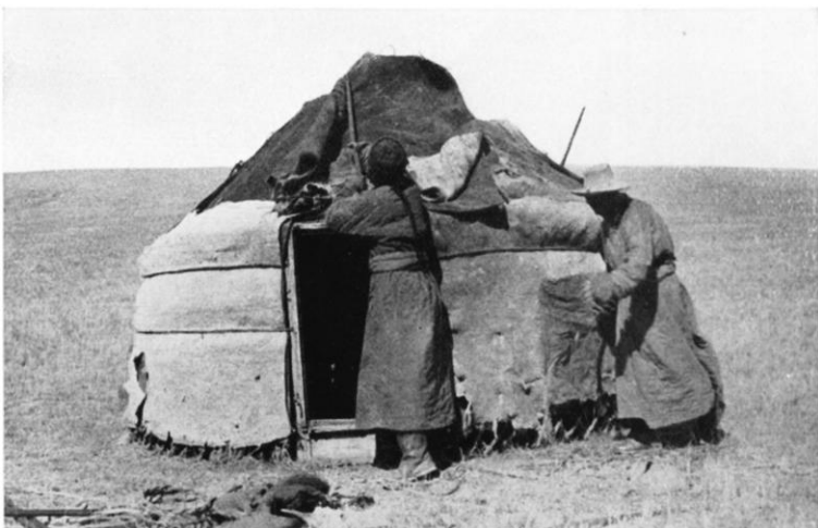
Adding the felt coverings to the framework of the tent
