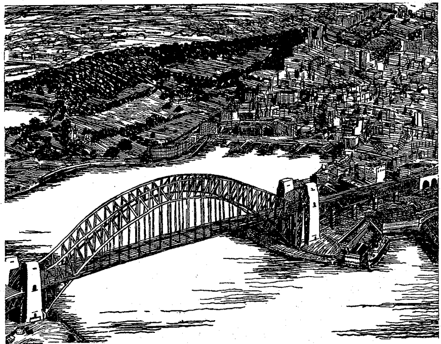
THE HARBOUR BRIDGE
