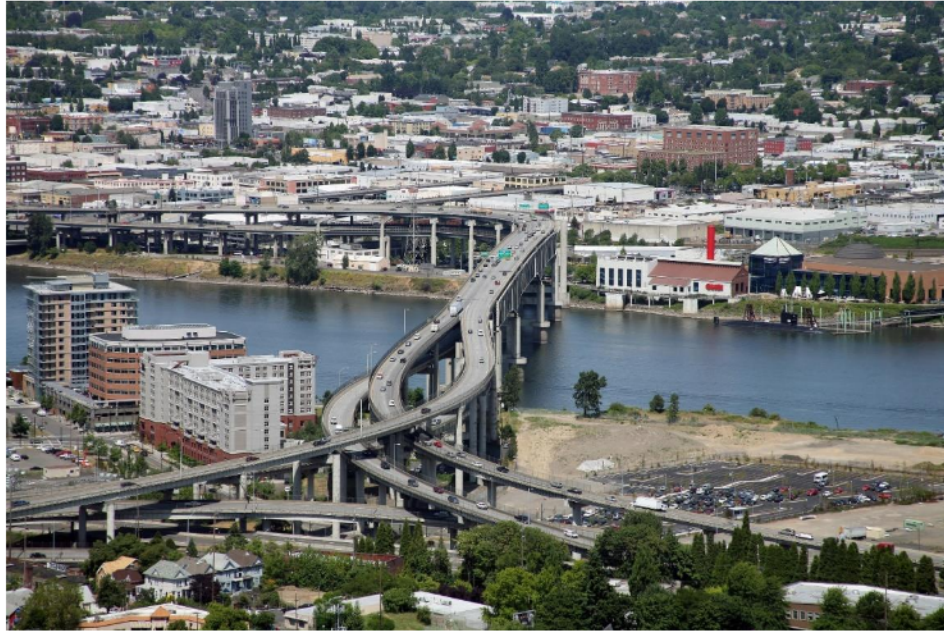
Marquam Bridge, Portland OR
